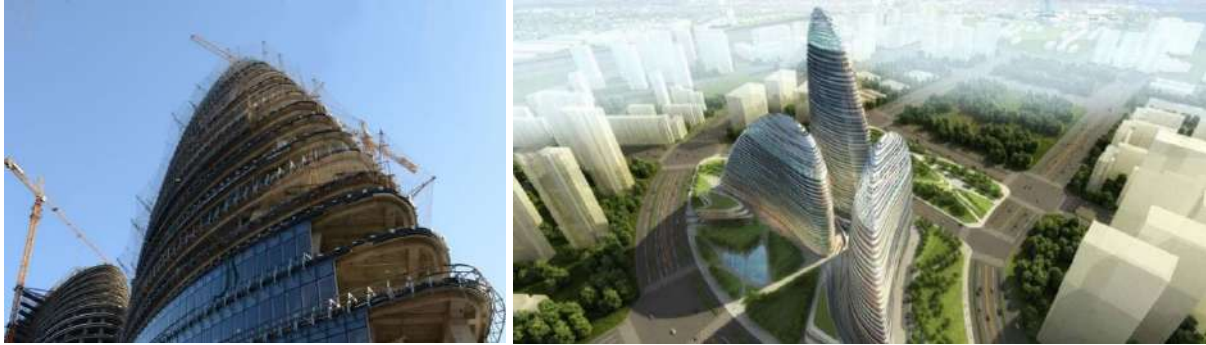
Figure 39 and Figure 40. Wangjing Soho Construction and Silhouette View, Zaha Hadid Architects, Shanghai, China (URL 19, URL 20)
